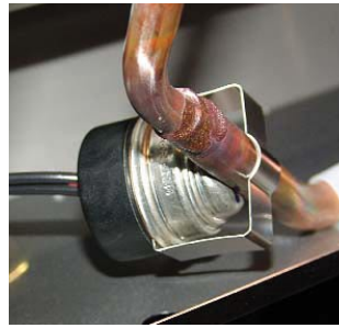
Figure 6: Defrost thermostat
