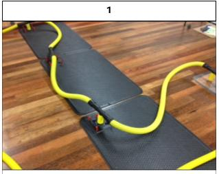
Before placing the Vac-It Panels onto the surface to be dried, remove all standing water. Place Panels onto the surface but do not place tape on the Panels at this time.
