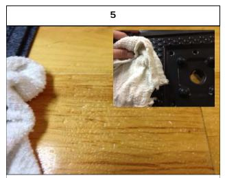
Now extract the floor for at least 30 minutes. Lift the panels occasionally to wipe away any visible liquid that may have pooled under the panels (on bottom of panel and on top of flooring). Extract until there is no more bulk liquid coming from flooring.
