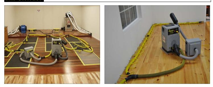
Injectidry's High Pressure drying systems are specifically developed to target high risk areas of hidden moisture such as: walls and ceilings, even those coated with watertight finishes like PVA paint and vinyl wallpaper coverings, double-sheeted fire walls, party walls, sound barriers, insulation, walls behind cabinets and fixtures and floors.
