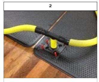
Attach the Panel T's or tubing from manifolds to the main drying lines.
